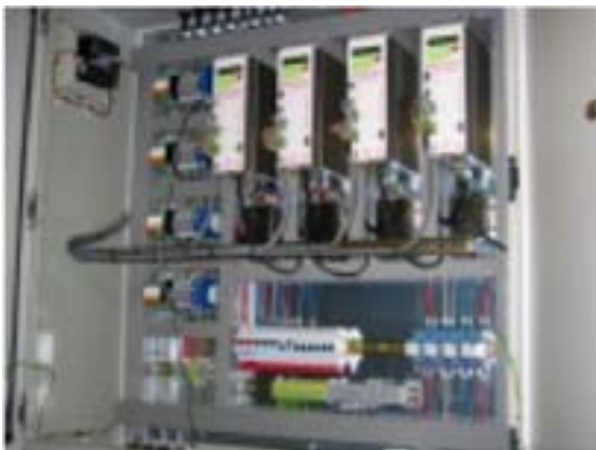
Drive electronics DACS2000 in remote explosion-proof enclosure
